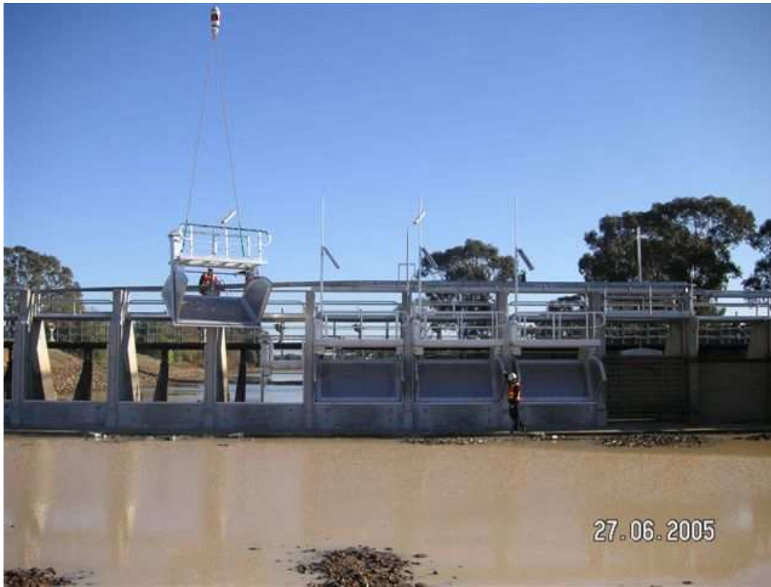
Photo 5: Rubicon gates under construction.
