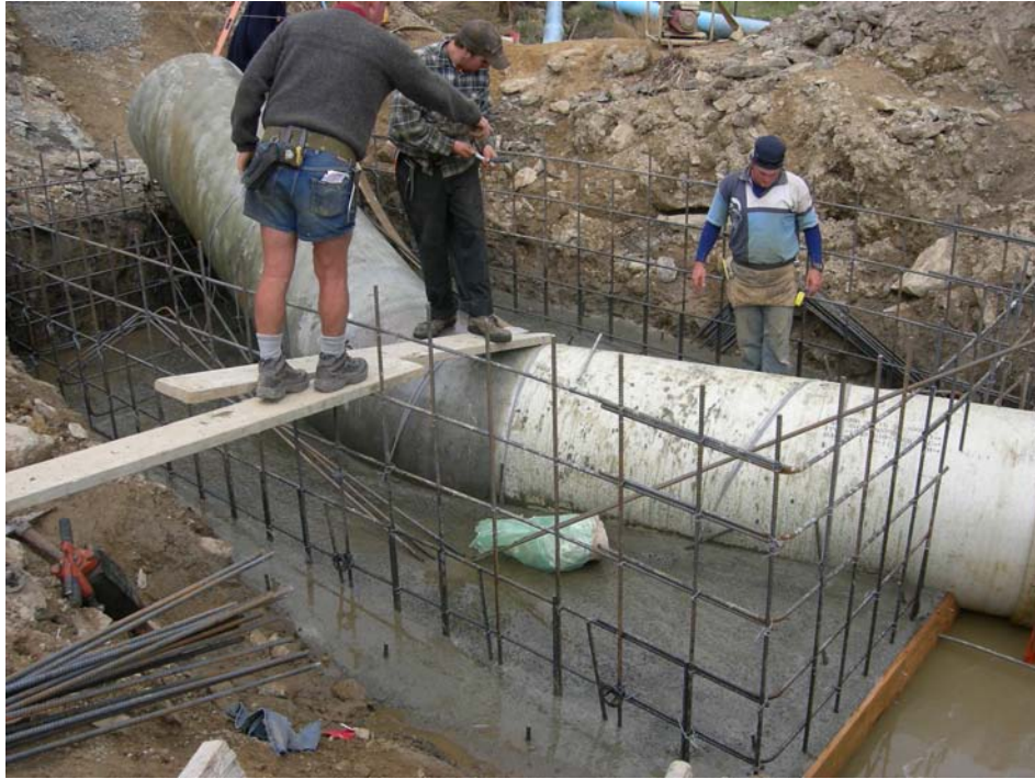
Photo 3: An FRP anchor block under construction (2007).
