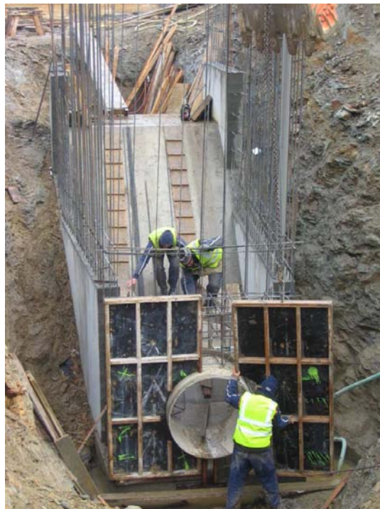
Photo 1: Example of a typical primary headrace canal offtake structure under construction (2007)
