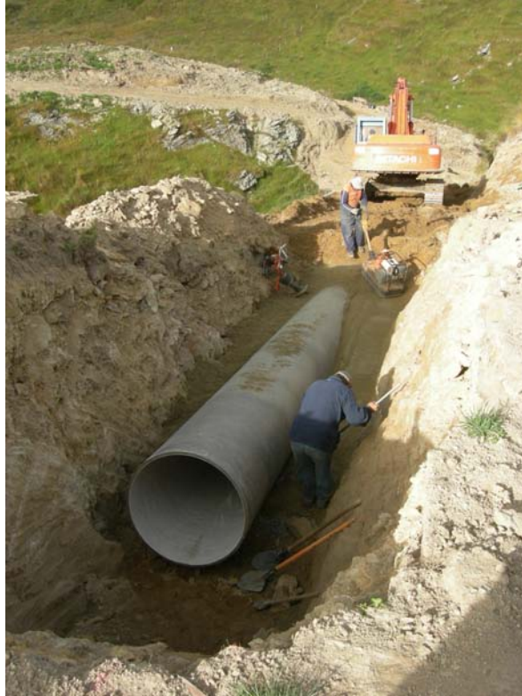
Photo 2: 1.1 m diameter FRP pipe (under construction 2007).
