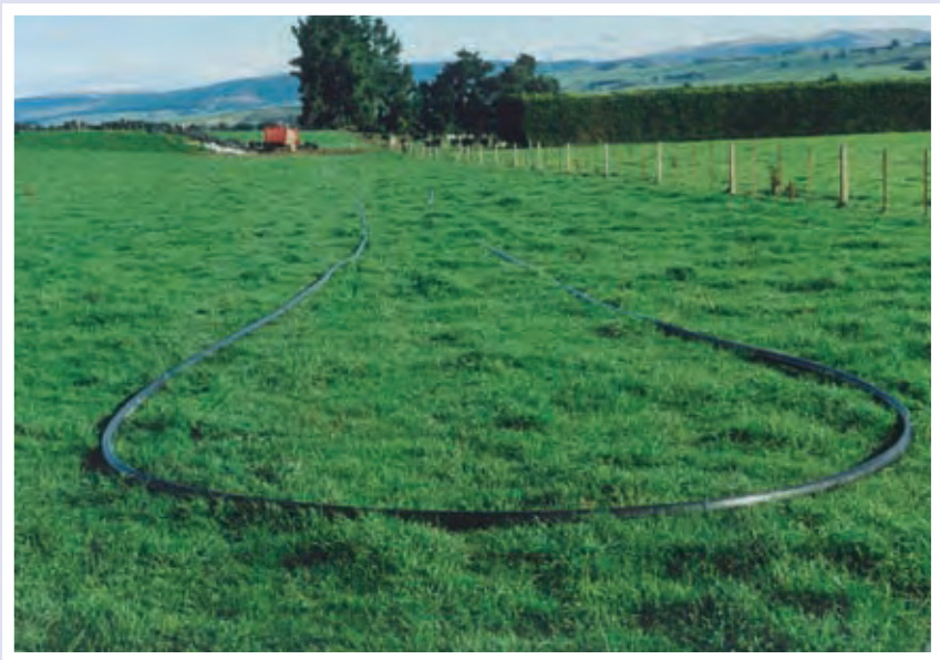
Pipe layout behind irrigator - Photo courtesy Otago Regional Council
