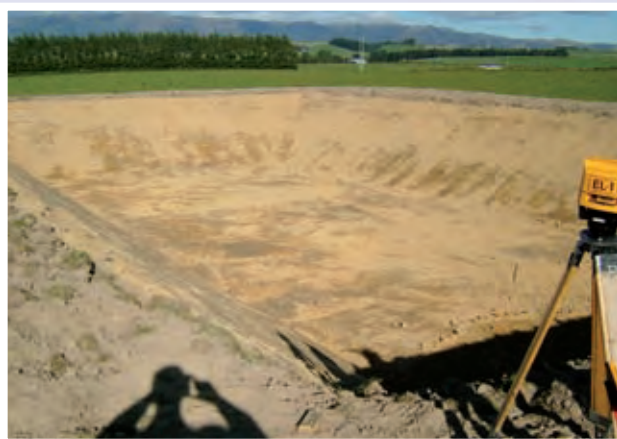
Recently constructed storage pond Photo Courtesy Scandrett Rural
