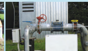
Meter too close to flange and gate valve, and insufficient straight length of pipe.
