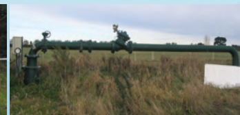
Meter too close to control valve and gate valve.
